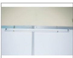
E2 日光灯 Fluorescent Lamp 220V/100W
